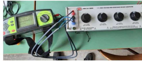
Figure 7. Test set-up in LEM for calibration of Metrel MI 2077 TeraOhm 5kV with the 5 kV IET Labs HRRSQ resistance reference standards decade
